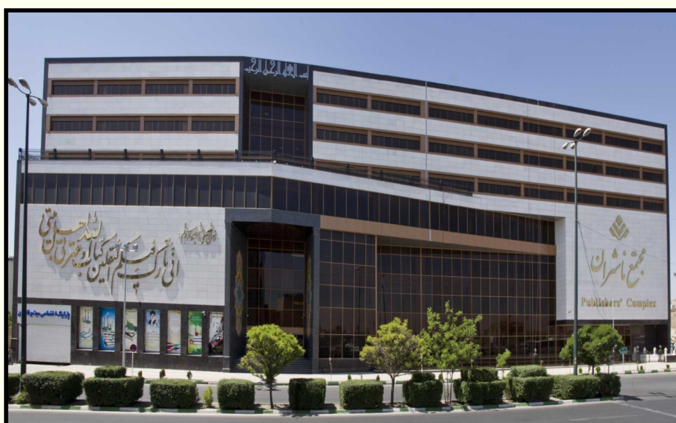
Outside View of the Seven Storey Publishers' Complex Building
